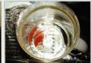
▲取付後に蛇口から出たサビのかけら After installing (rusted pieces are washed out).
